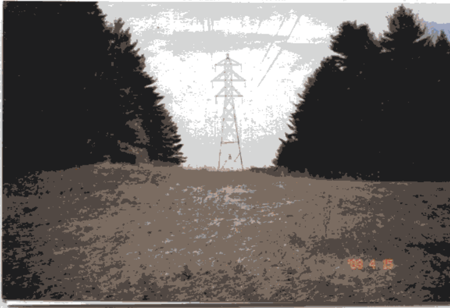
2.18 on powerline looking south
