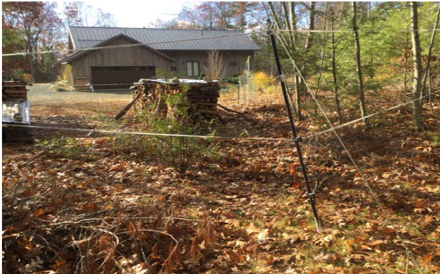
PHOTO 1: Boundary violation on north line of Matsuda. Pin 32 is presumed to be under wood pile. This situation has existed for many years.
