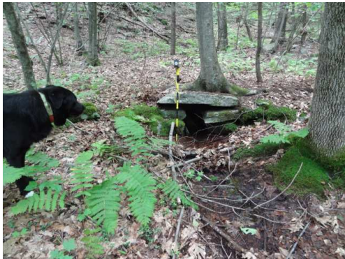
7. Stone structure covering spring
